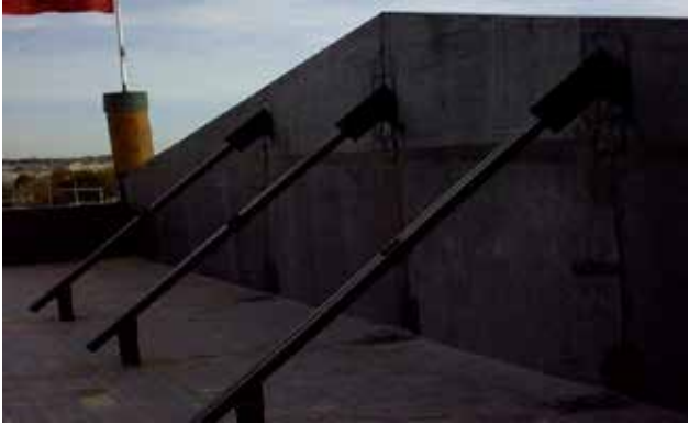
Paint diagonal roof bracing black.
