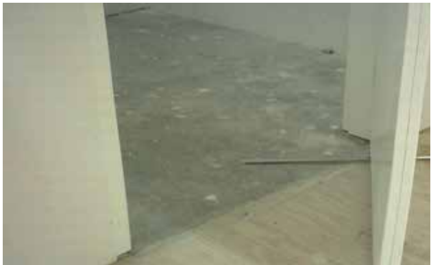
Slope concrete to meet plywood floor at mezzanine.
