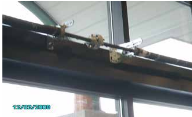
Example of how cart door springs and shaft mounting. Blocking installed prior to black anodized metal.
