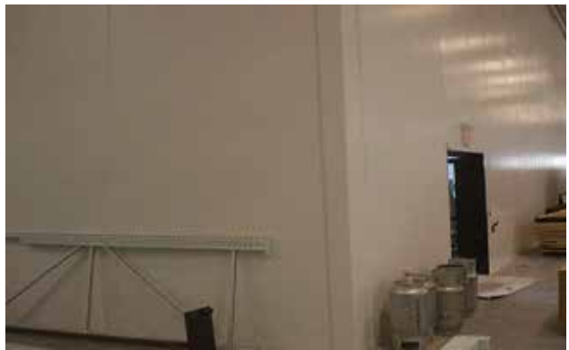
Caulk both sides of column to precast (2 locations) at receiving and paint to match walls.
