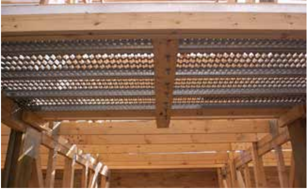
Board shed grip strut support with through bolts. Cut off bolt ends flush with nuts.
