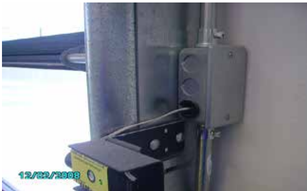
Example of photo eyes wiring hidden and tied.
