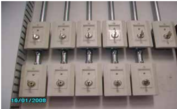
HVAC unit reset switches (to be labeled)
