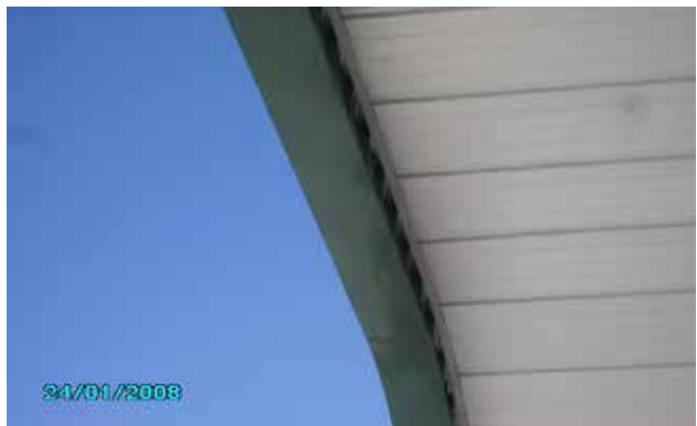
Specialty trim at exit and entrance – not fastened to the face.
