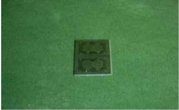
Typical quad box installation (with two outlet type covers) in carpet area.
