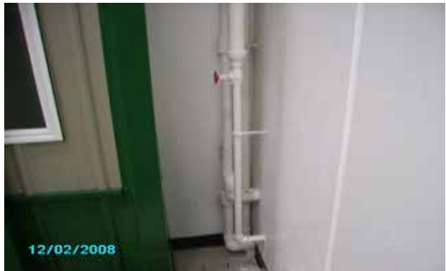
Example of sprinkler and plumbing drops in building materials by pole barn display within 8" of wall.
