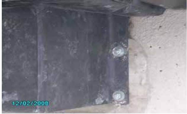
Example of expansion anchors (four per bumper)
