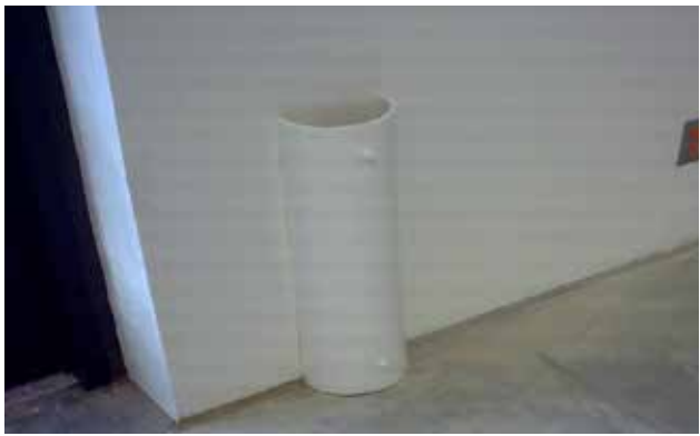
Install protective cover over plumbing for receiving area sill cock and paint.
