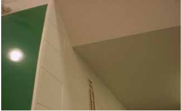
Front office area drywall ceiling with straight clean edges and caulked to walls with paintable caulking.
