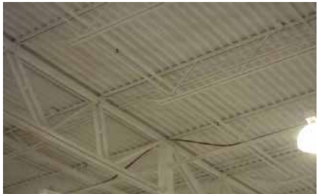
Correct run of low voltage wire over girder. Do not run joist to joist because of sagging.
