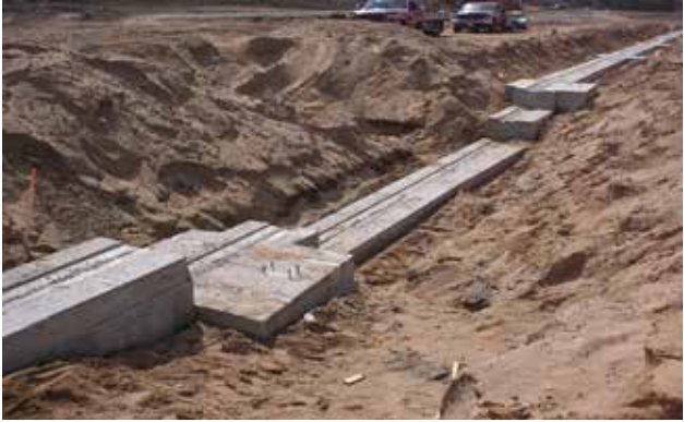
Typical perimeter footings with temporary shore anchor bolts and keyway on all 4 sides.
