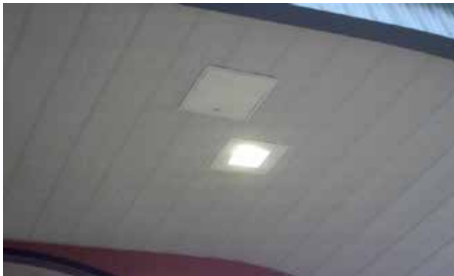
Example of front entrance soffit with access hatch and recessed light fixture.
