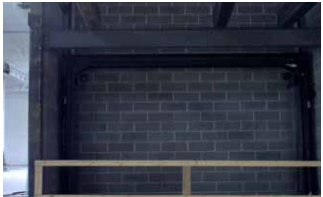
Elevator hoist way installed. Ready for mason to complete the openings.
