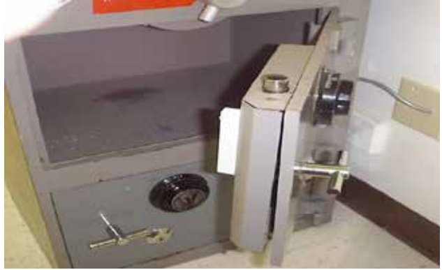
Safe door contact installation.
