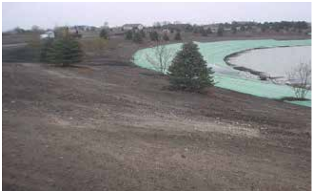
Example of acceptable final grade prep prior to seeding with smooth, level surfaces and nothing larger than 1/2" in diameter, No high and low spots.
