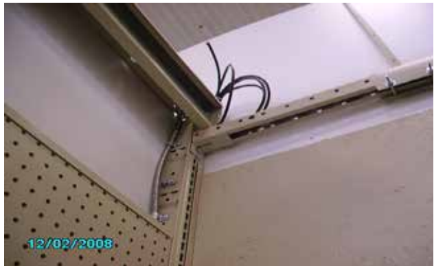
Coax wiring for department monitors.
