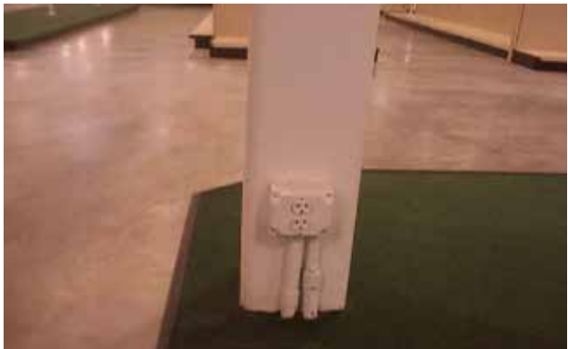
Typical outlet on column installation painted white to match.
