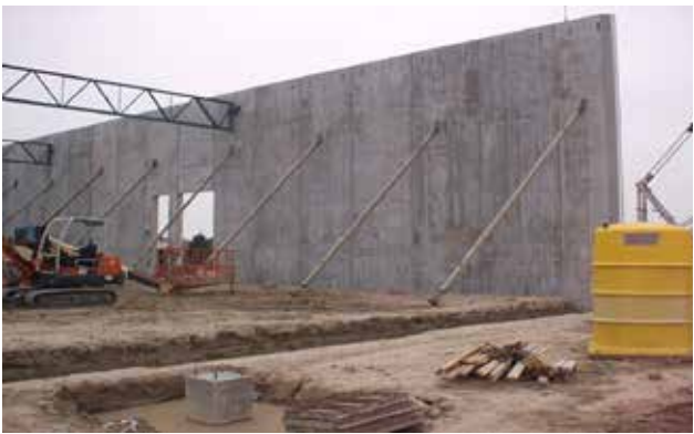
Example of helical anchor free-stand method of precast panel installation.
