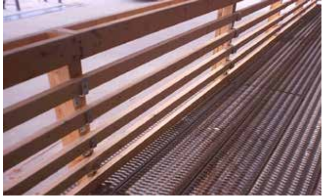
Complete treated board shed catwalk & Railings.
