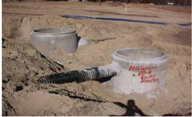
Typical manhole with piping penetrations sealed with concrete (as required per civil drawings/local authorities)
