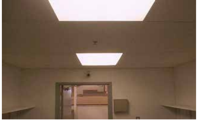
Typical drop ceiling with recessed lights. Track tight to walls and level throughout.
