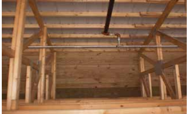
Treated board shed dry sprinkler system must not interfere with lumber product.
