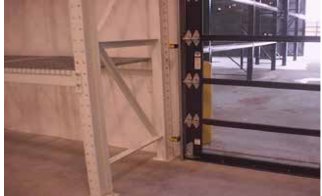
2 sets of photo eyes set 1' and 5' A.F.F.
