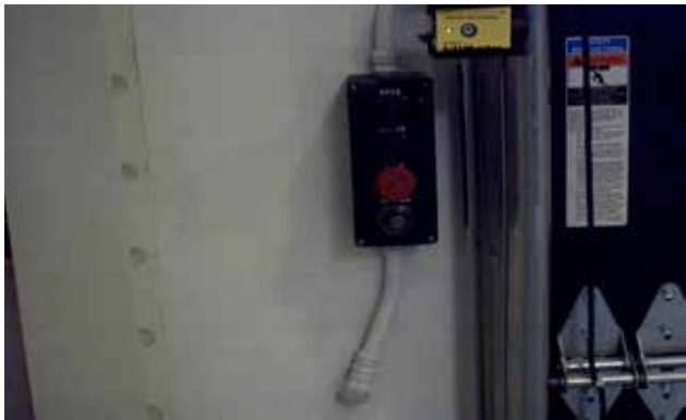
Example of overhead door buttons with key switch to shut off operator.
