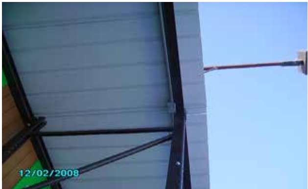
Electrical example for pallet rack lights.
