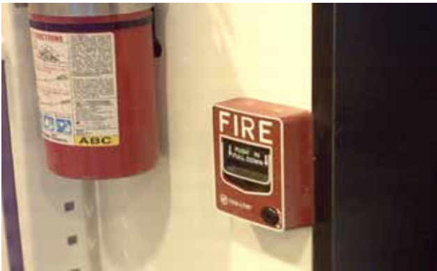
Pull station. This always needs to be installed this close to the door.
