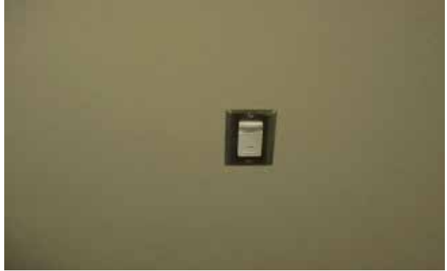
Typical motion sensor light switch with stainless steel cover plate.
