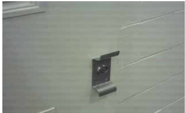
Example of exterior pull handle to panic bar hardware at electrical room doors and elevator mechanical room door.
