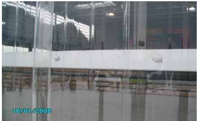
Clear panels always fastened in the flats.
