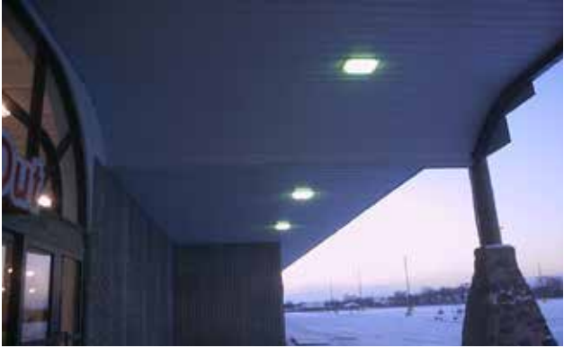
Example of front canopy soffit and exit canopy rolled soffit.
