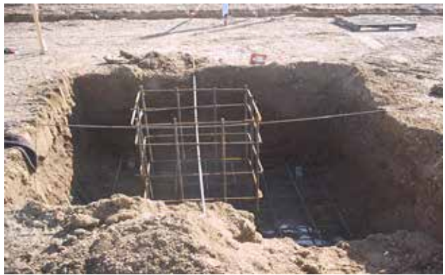
Typical footings and piers rebar installation.
