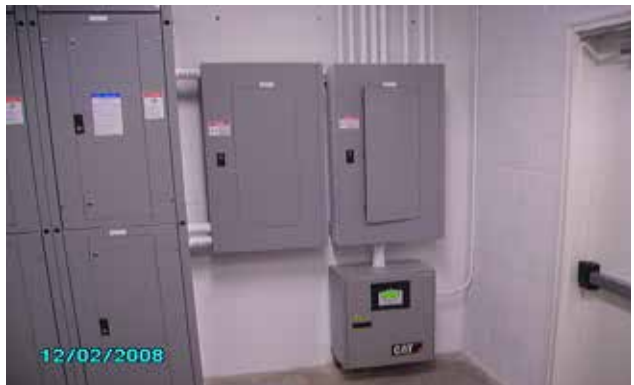
Example of separate generator panels.
