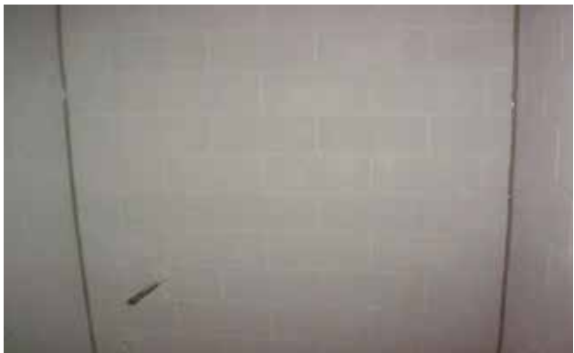
Typical masonry to masonry caulk joint completed prior to final coat of paint.
