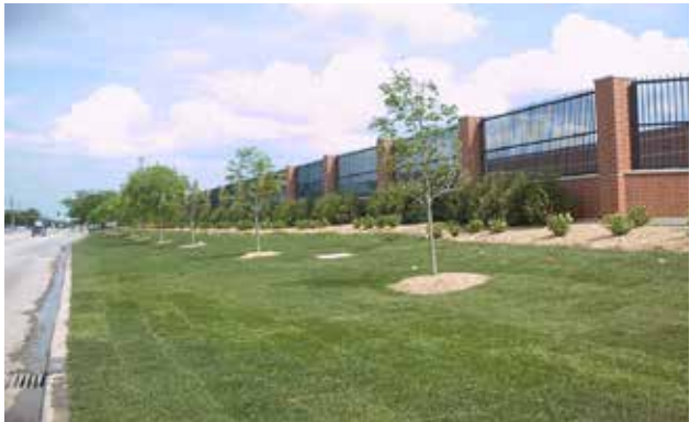
Example of sodded area with no high and low spots. No gaps between sod roll joints. Trees to be tied off per plan and specifications until established.
