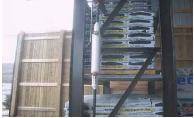
Example of drum drip with heat tape and power for freeze up protection.
