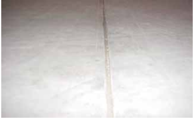
Polyurethane control joint & construction joint caulking – no residue on slab.
