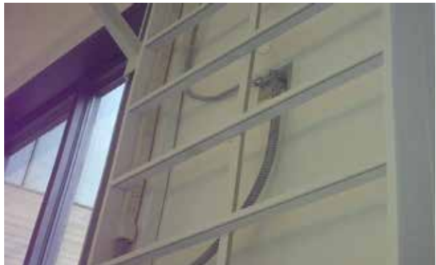
Example of Electrical department wall cloud wiring/plugmold.
