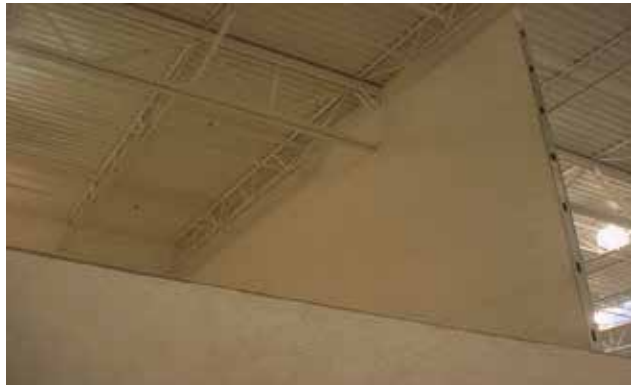
Interior mezzanine walls complete – filled in around all penetrations, etc.
