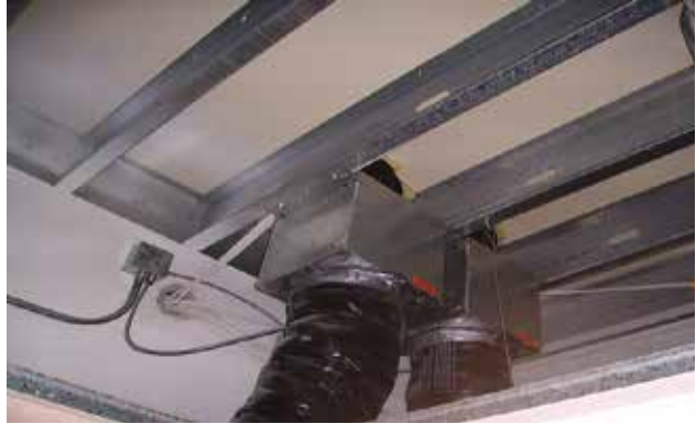
Example of exhaust fans in monitor room.
