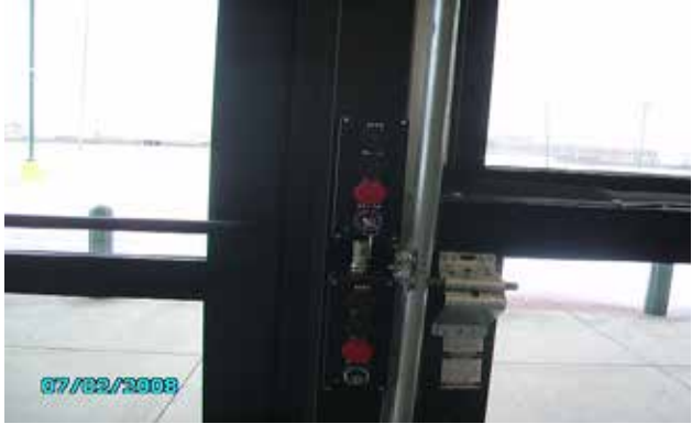
Example of two sets of keyed switches at cart doors
