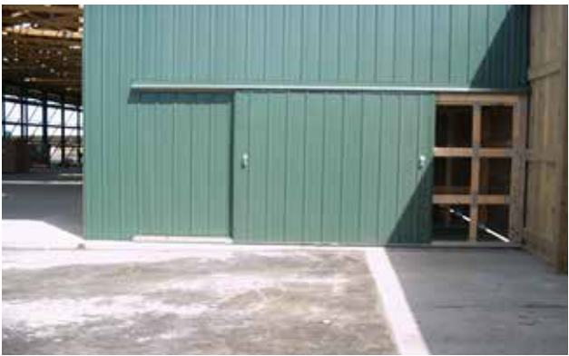
Sliding door on treated board warehouse.
