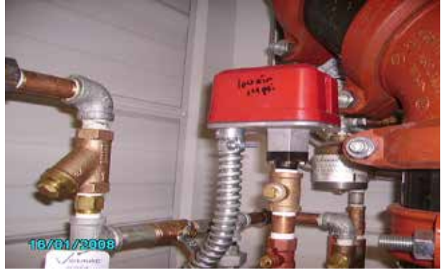
Low air switch in warehouse.
