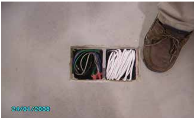
Example of completed floor box – cut out per spec.
