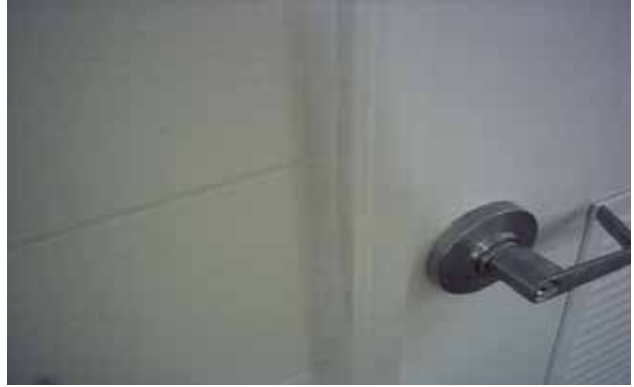
Example of brick mold caulked to masonry walls with straight/clean paint cut line.
