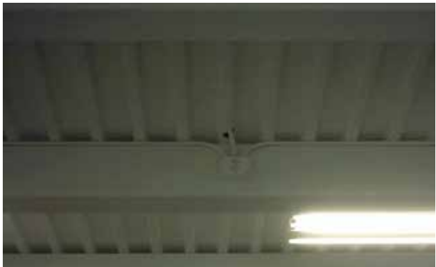
Example of outlets of Hardware mezzanine. Conduits tight to deck. In deck flutes whenever possible.
