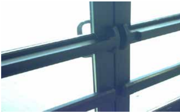
Example of double man doors with panic push bars and rubber bumpers.
