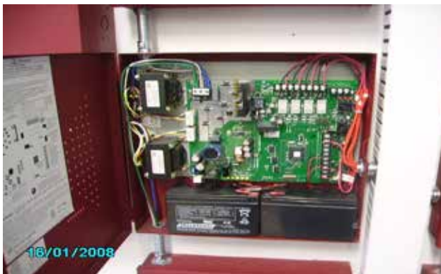
Neatly wired fire/security panels.
