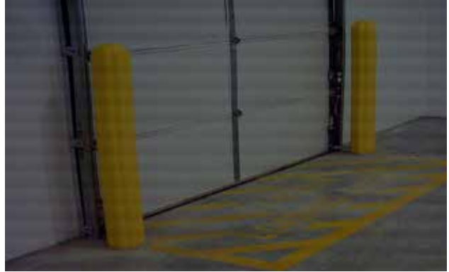
Install yellow bollard covers. Trim to length as required.
