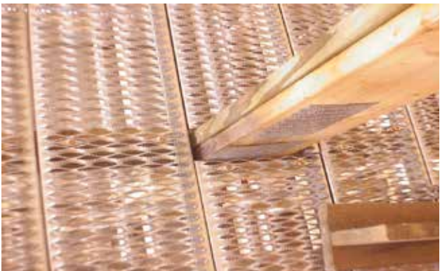
Grip strut cut around racking leg and thru-bolted into 2x member.
