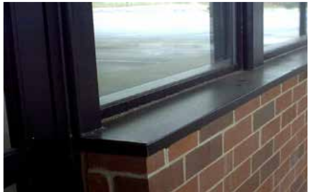
Example of black anodized cap at garden center wall.
