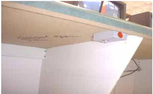
Installation of emergency alarm at front office.
