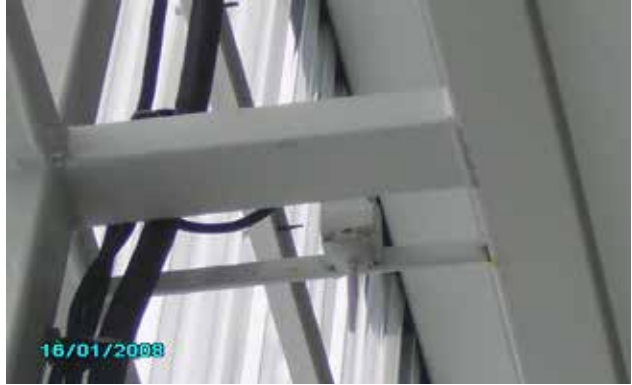
Bi-fold door limit switch (center of door)
