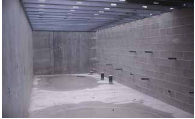
Typical completed masonry plumbing wall in bathroom location. Plumbing as required per fixtures – verify.
