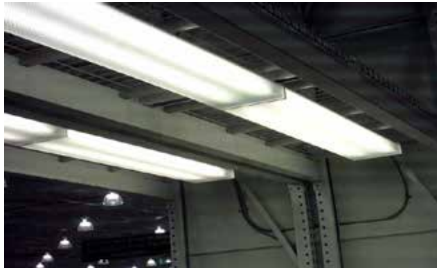
Example of fluorescent lighting in pallet racks.
