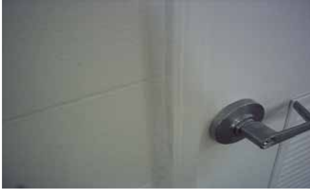
Example of brick mold caulked to masonry walls with straight/clean paint cut lines.
