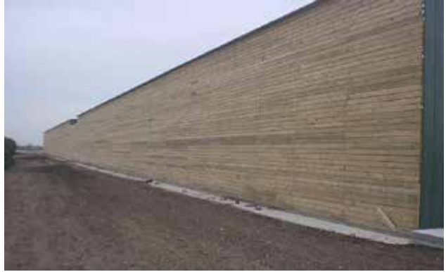
Example of tongue and groove back wall of treated board warehouse.
