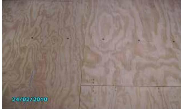
Straight screw pattern on mezzanine deck and tight joints.
