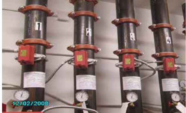
Complete flow switches.
