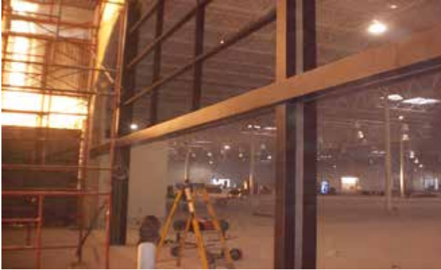
Example of black anodized break metal installed at front entrance per plan.
