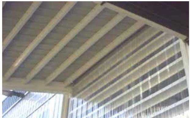
Example of clear panels and girts above garden center overhead doors.
