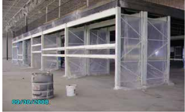
Example of hardware mezzanine paint masking on racks.
