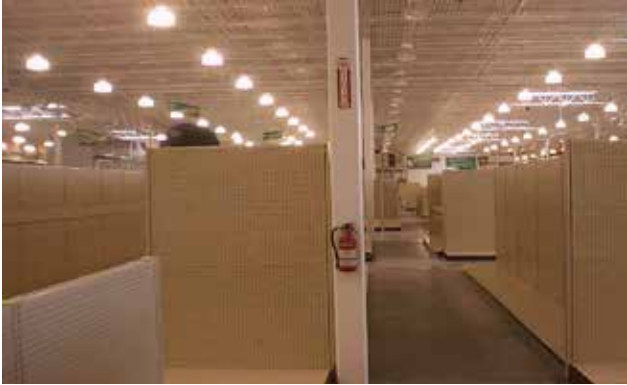
Typical fire extinguisher to column installation (sign by others) Verify height with local authority prior to installation.
