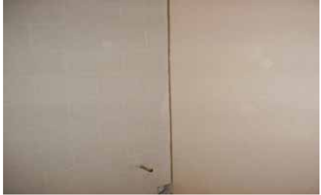
Typical masonry to precast caulk joint prior to final painting.
