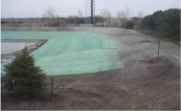
Example of erosion mat on 3 to 1 slope (or greater) and hydro-seed placed on acceptable final grade.
