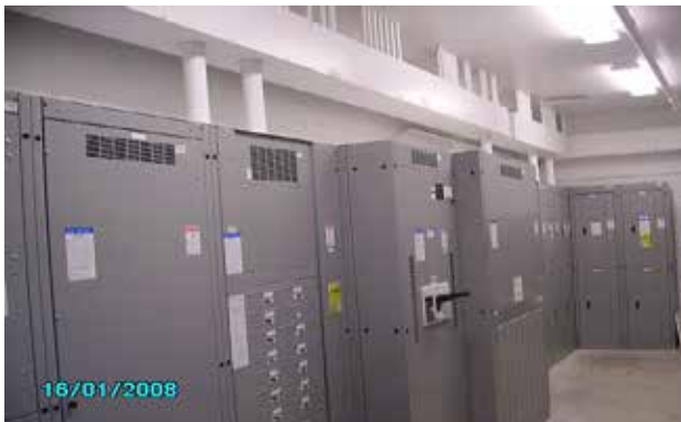
Example of switch gear.
