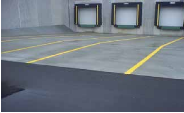
Dock levelers, bumpers (4 expansion anchors per bumper required) and cushions. See manufacturer's recommendations for installation.
