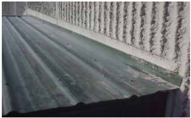
Trim saw cut into precast with caulking.
