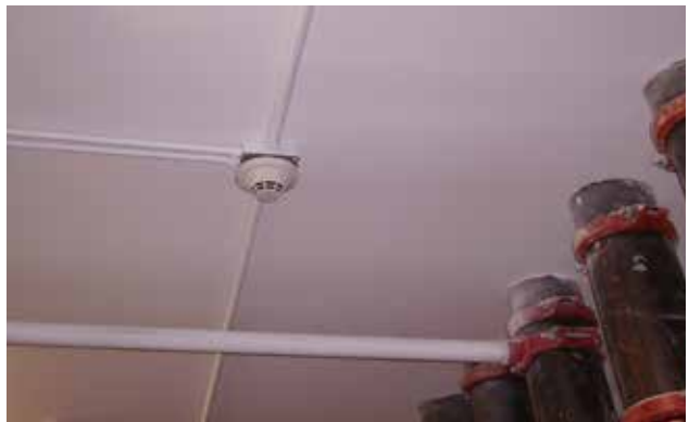
Sprinkler room smoke detector.
