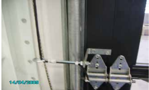
Example of coil cord wire – eyebolt.
