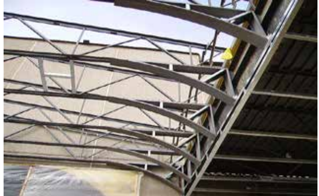
Example of exit canopy truss construction with light gauge radius frames.
