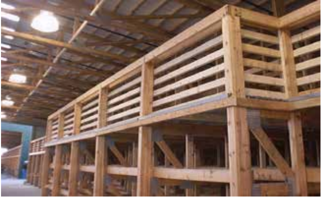
Completed treated board shed catwalk & railing.
