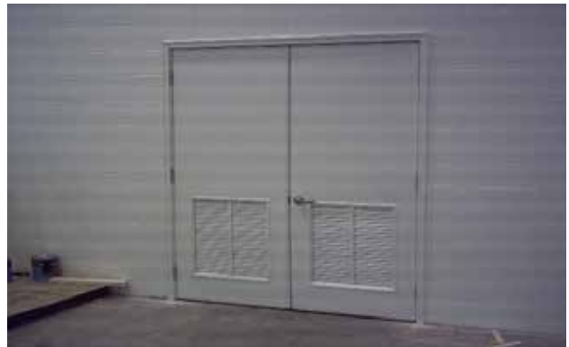
Example of janitors room doors with passage style door handle and no closures, painted white.
