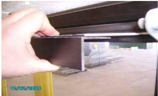
Example of angle to be installed on 16' wide overhead door.
