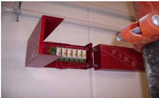
Module boxes in main sprinkler room.
