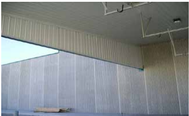
Example of attached guard shack soffit steel.
