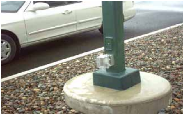
Example of outlet on light pole.
