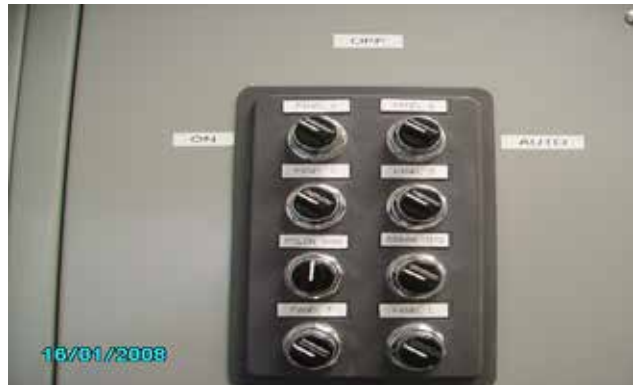
Integrated by-pass switches.
