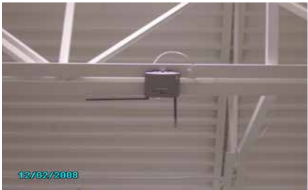
Overhead CAT 5 for computer location.
