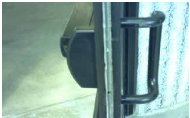
Example of man door panic push bar and exterior pull handle.
