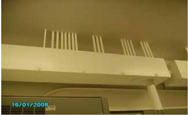
Acceptable drops and raceway to switch gear or as required by code.
