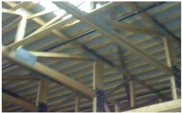
Splice plates at warehouse trusses.
