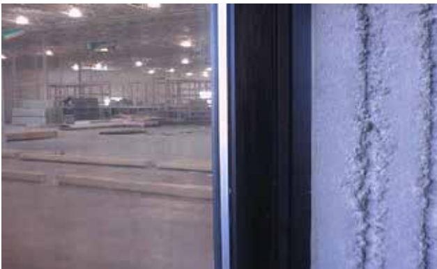
Continuous hinge on all single and double man doors.
