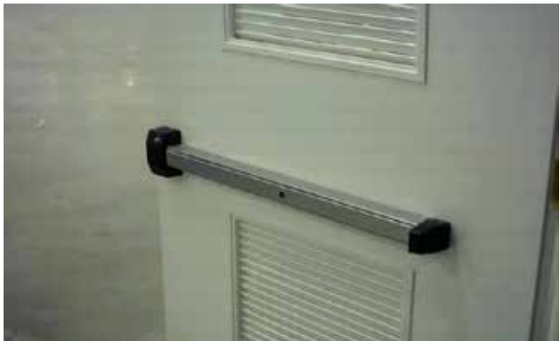
Example of large electrical room door panic bar.
