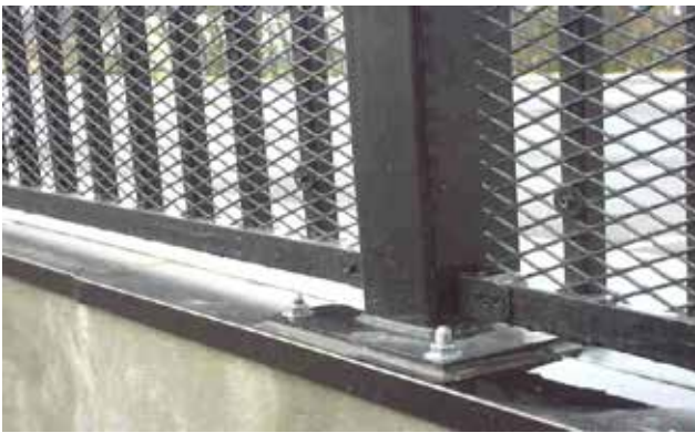
Wrought iron fence complete with stainless steel anchor bolts.
