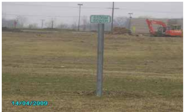
Example of utility marker with metal stake and sign.
