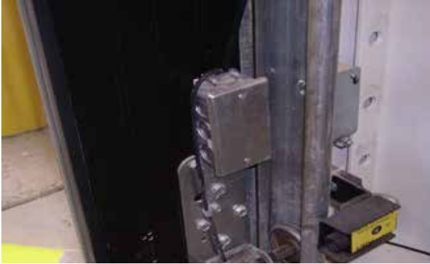
Example of acceptable “J” box mounted on door for cord coil to miller edge connector.
