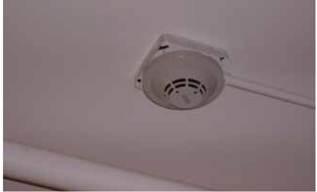
Example of smoke detector.
