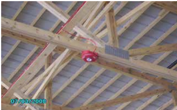
Example of weatherproof warehouse horn strobe (if applicable)
