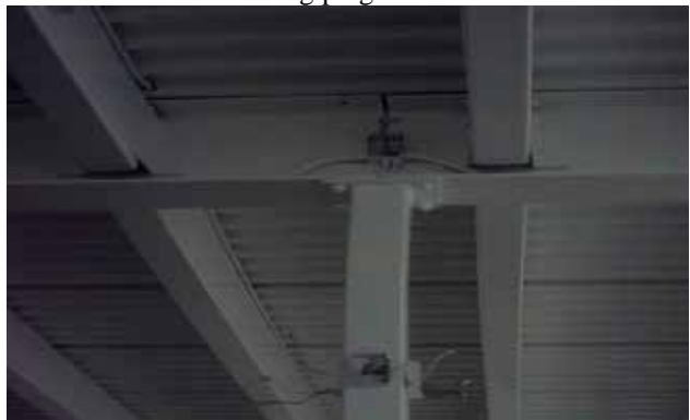
Example of column light electrical. Flex through bearing plate into column.
