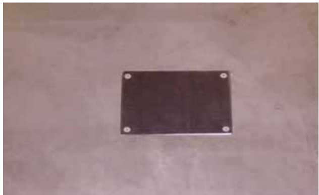
Example of recessed stainless steel cover plat for abandoned/relocated floor box (two gang shown)
