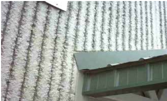
Example of canopy flashing precast riglet cut and caulked.
