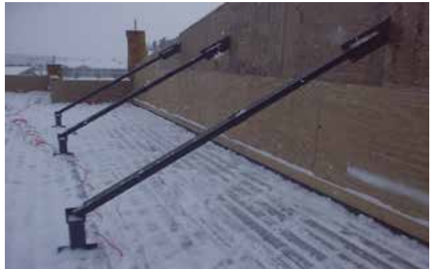
Front canopy parapet bracing.
