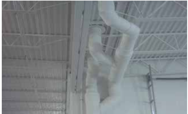
Example of acceptable interior drain piping in receiving area.
