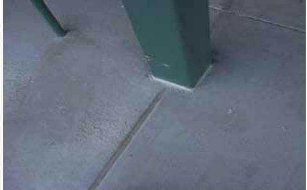
Caulking around exterior columns to concrete.
