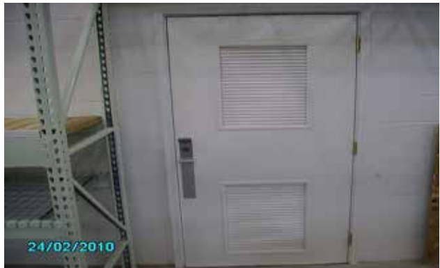
Large electrical room door with two louvers.
