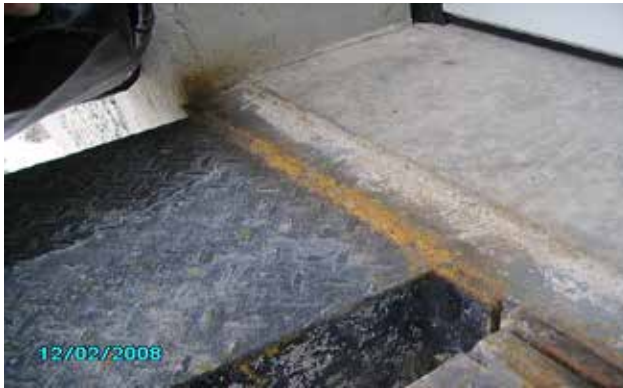
Example of full welds on bumpers and levelers.
