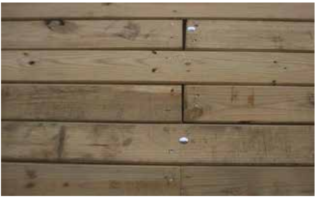
Example of through bolts and stainless steel fasteners on back wall of treated board warehouse.
