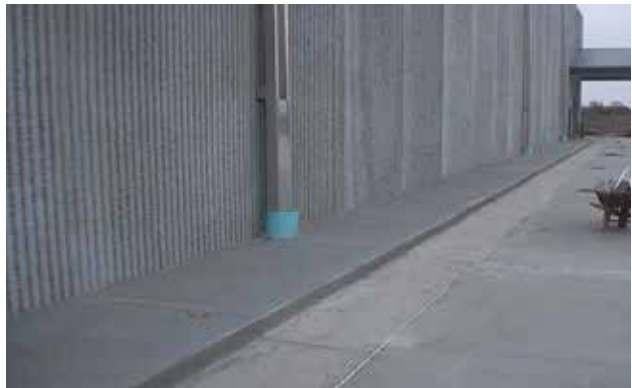
Example of downspout storm with bell end flush to pallet rack slab and 1' PVC sleeve above grade.
