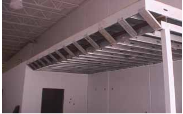
Typical light gauge framing at front office area.
