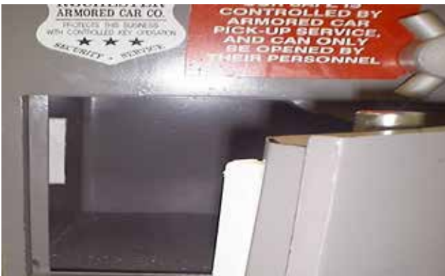
Safe door contact installation.
