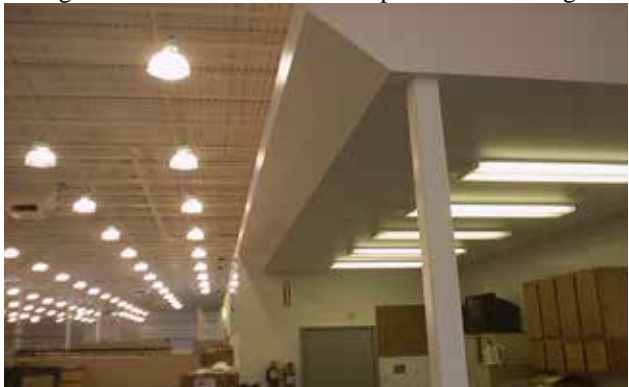
Front office area drywall ceiling with straight clean edges.
