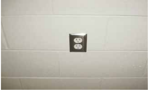
Typical outlet. Recessed with stainless steel cover plate.
