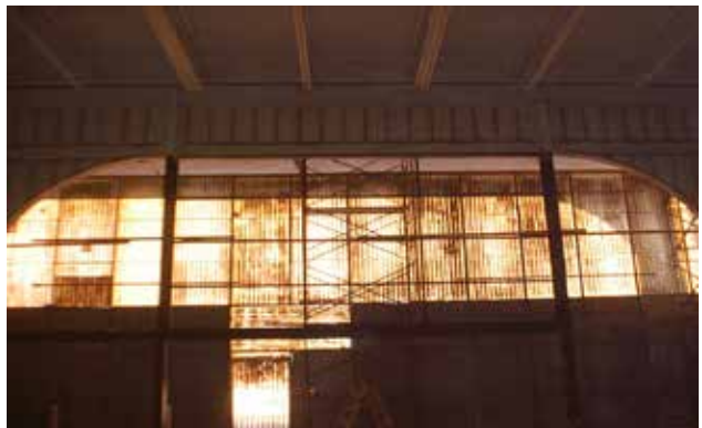
Front entrance insulation and vapor barrier ready for drywall.
