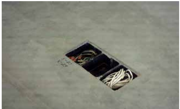
Example of complete wire pulls ready for fixturing phase. Concrete cut straight and no more than 1/4" cut out around box.
