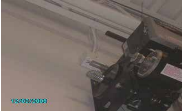
Disconnect switch at overhead door operators.
