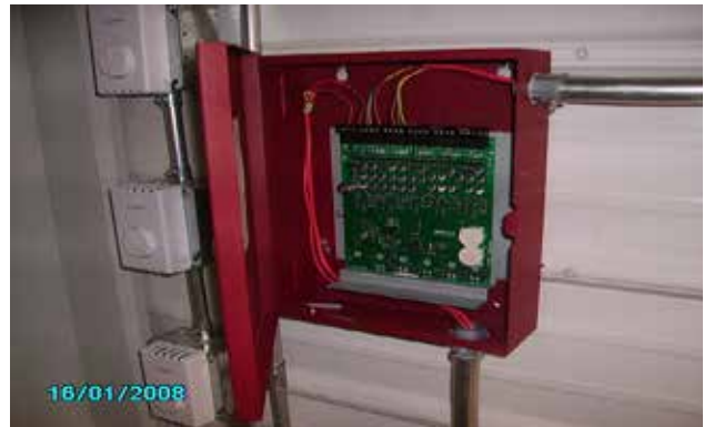
Warehouse panel wired neatly.
