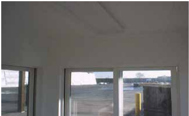
All joints, corners, door jambs, thresholds, etc., caulk with paintable caulk prior to painting in guard shack (no voids)
