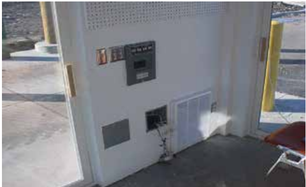
Electrical at guard shack with push button and stainless steel cover plates.
