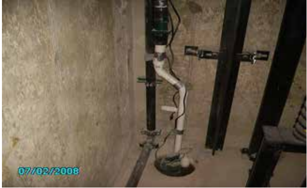
Example of sump pump in elevator.
