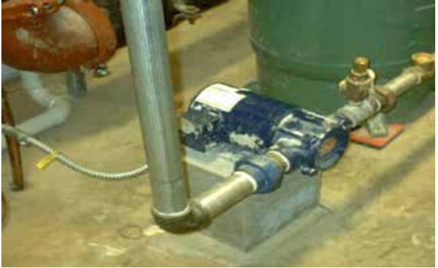
Jockey pump pad. Concrete poured by General Contractor if required.
