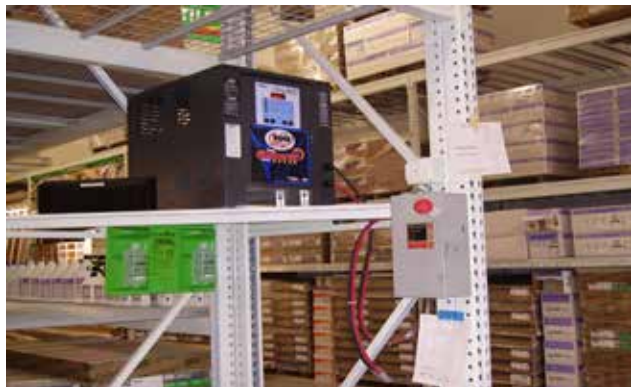
Battery charger and disconnect.
