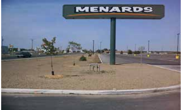
Example of seeded area. Fine graded with no rocks, dirt clumps, etc. larger than 1/2" diameter. Trees are mulched, tied off plumb and plastic protection installed. Low and high spots in grades leveled for final appearance.
