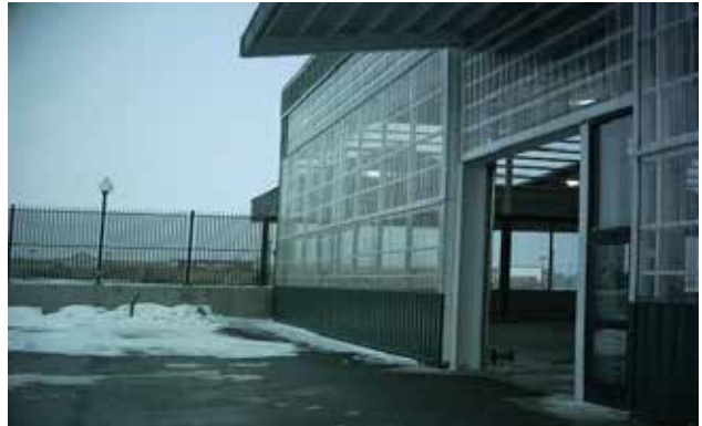
Example of bi-fold doors complete with painting, sheeting, operators, etc.
