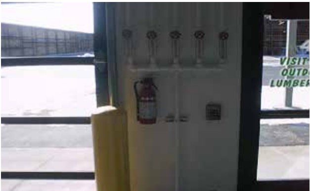
Example of painted sprinkler drops between doors 3 & 4 with appropriate metal signage.
