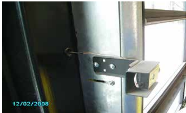
Example of photo eyes wiring hidden and tied.
