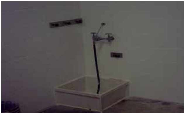
Mop sink with mop hangers, faucet and hose. Caulk around entire sink to floor and wall.
