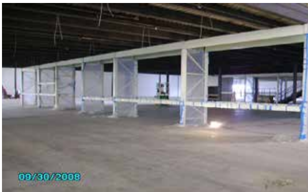
Example of masking off racking. Note: The cut line below structural rack beams.
