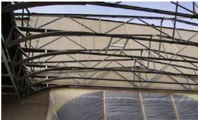
Example of exit canopy truss construction.
