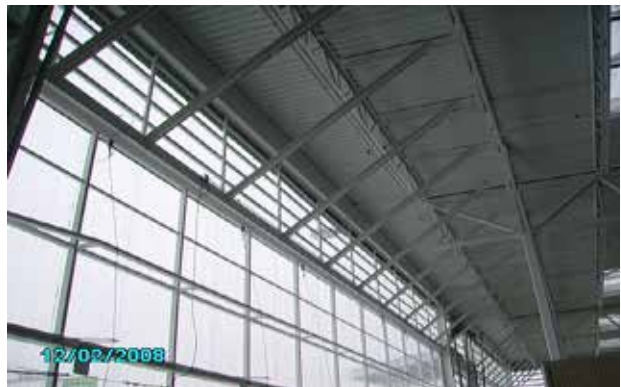
Example of bi-fold door structural steel.
