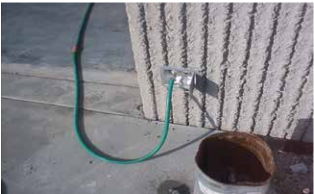
Exterior flush mounted sill cock. Caulked all four sides for complete installation.
