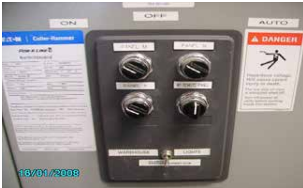
Integrated by-pass switches.
