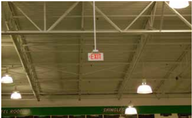
Example of acceptable exit sign in retail area mounted on rigid conduit (painted white). Mounted at AHJ approved height if mounting in bar joists is not acceptable.
