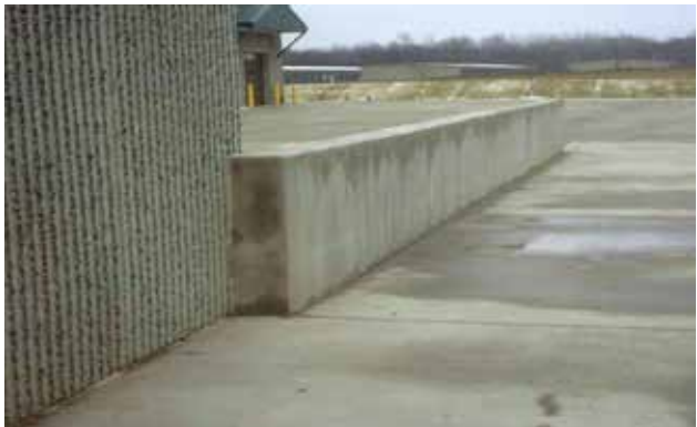
Rub out loading dock retaining wall.
