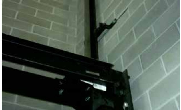
Example of hoist way and imbeds.
