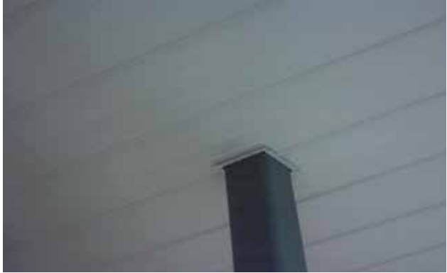
"J" trim at soffit around columns.
