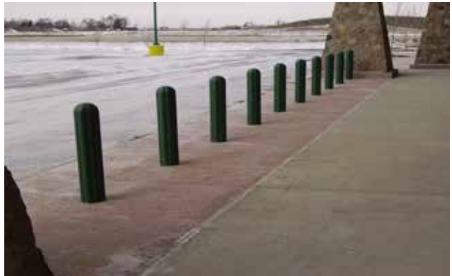
3' bollard covers at entrance, glued and caulked.
