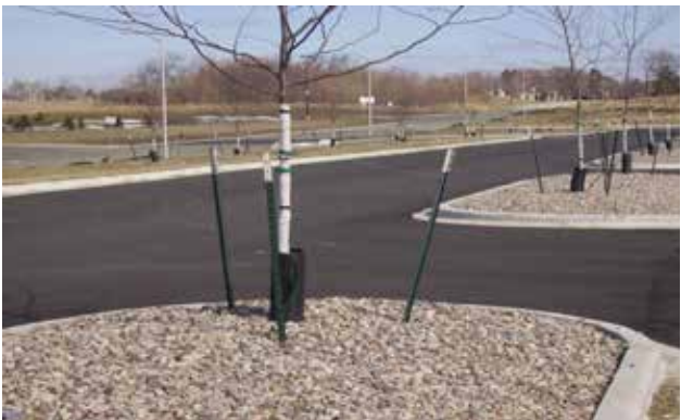
Example of island trees with staked, tree wrap and drain tile per plan.
