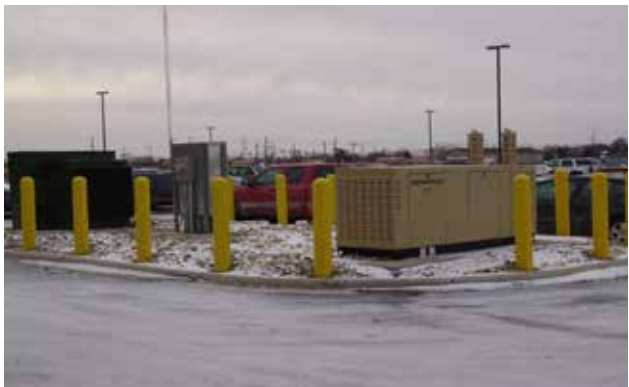
Generator, CT cabinet and transformer island.
