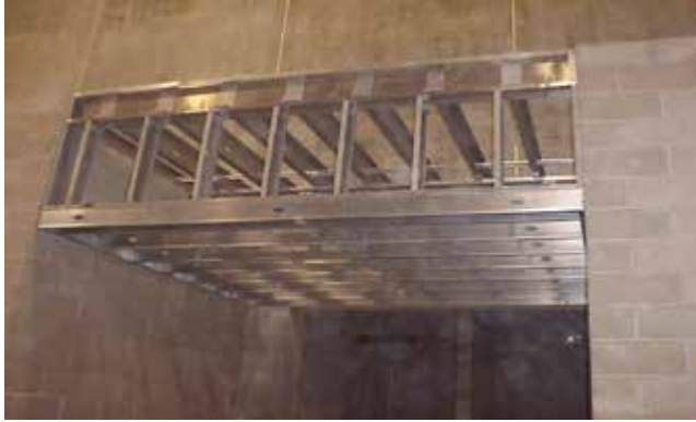
Typical hallway light gauge framing.
