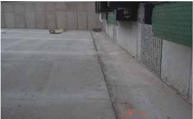
Example of receiving swale to storm inlet/grate for proper drainage.
