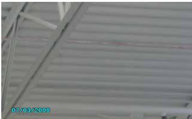
Fire/burg wires ran on top of bottom cord and wind bracing to be hidden as best as possible.
