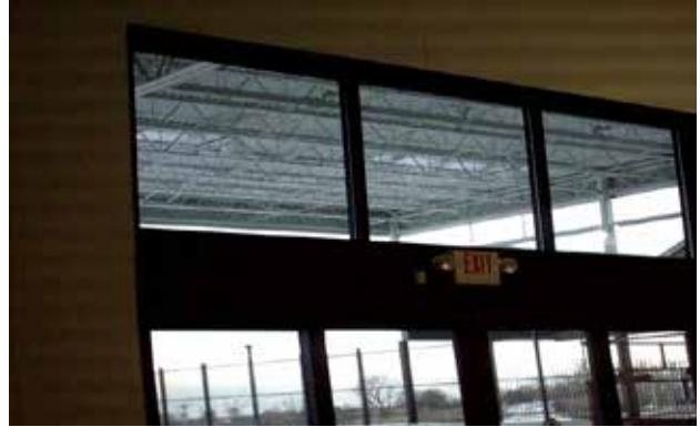
Wrap all jambs and headers with black anodized break metal. Note: Also wrap beam connection plate. Caulk all break metal to frames (black).
